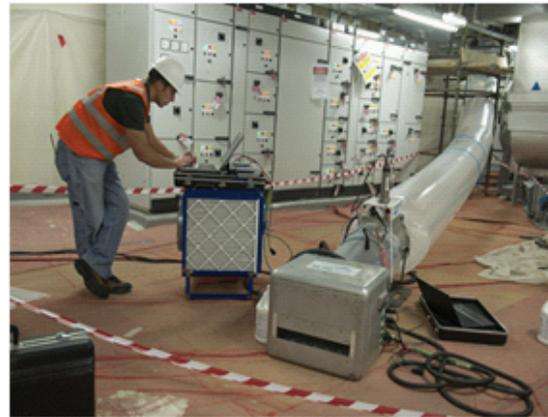
**Goals:** Building engineers used AeroSeal with the following goals in mind: *Reduce leakage to more than 8%. Seal leaks without disrupting new construction. Attain LEED Gold certification. Meet schedule for construction completion date.*
