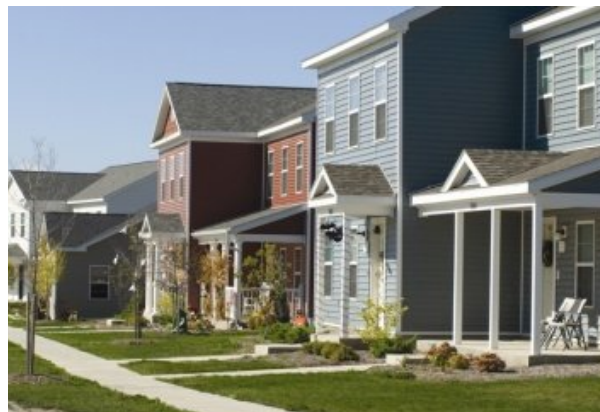
Fort Drum Mountain Community Homes: 3,600 Energy Star® Certified Homes.
